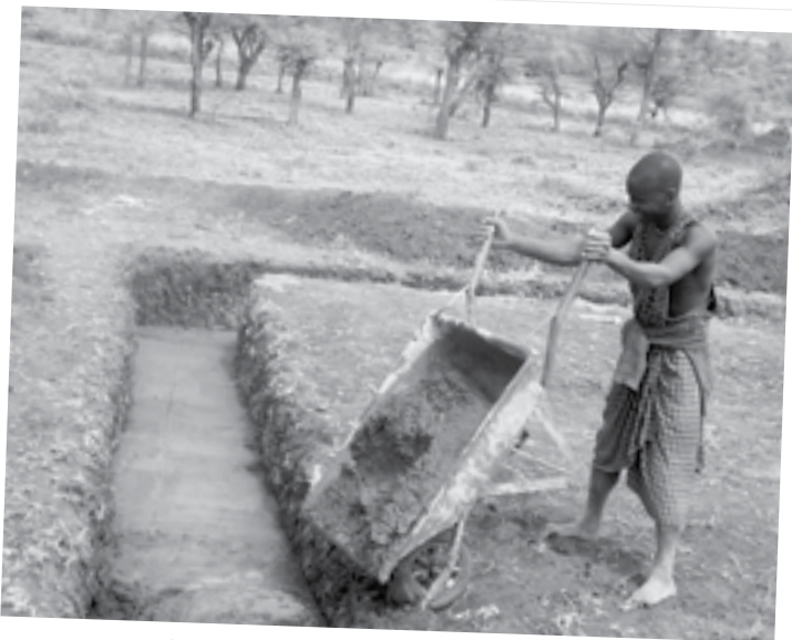
New church building foundation.
