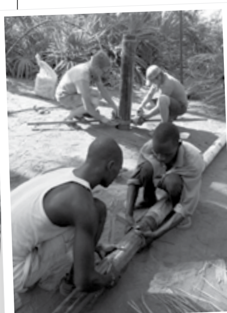
Interns casing a well.
